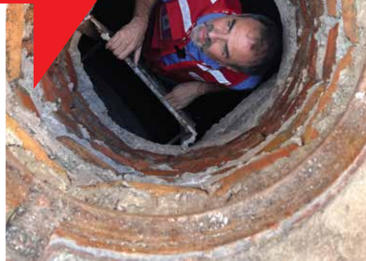
In Cherkasy, Ukraine Canadian Red Cross Shelter Coordinator, Rodolfo Magirena inspects pipes in the Regional Children's Hospital that have become corroded and are no longer able to efficiently pump heat into the building.
