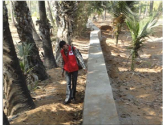
Flood diversion wall constructed under CBDRR mitigation activities
